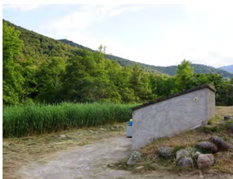
Station de phytoépuration
